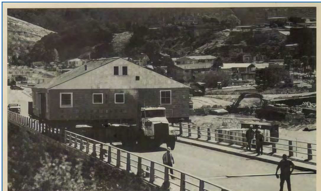
San Luis Yacht Club move. Moving the Yacht Club was complicated by its width, which is greater than the bridge over which it had to travel on its way to a temporary berth at Cherry Canyon. Experienced professionals had some anxious moments until the flatbed truck made it past the barrier without mishap. © Dale Reid Ginder
